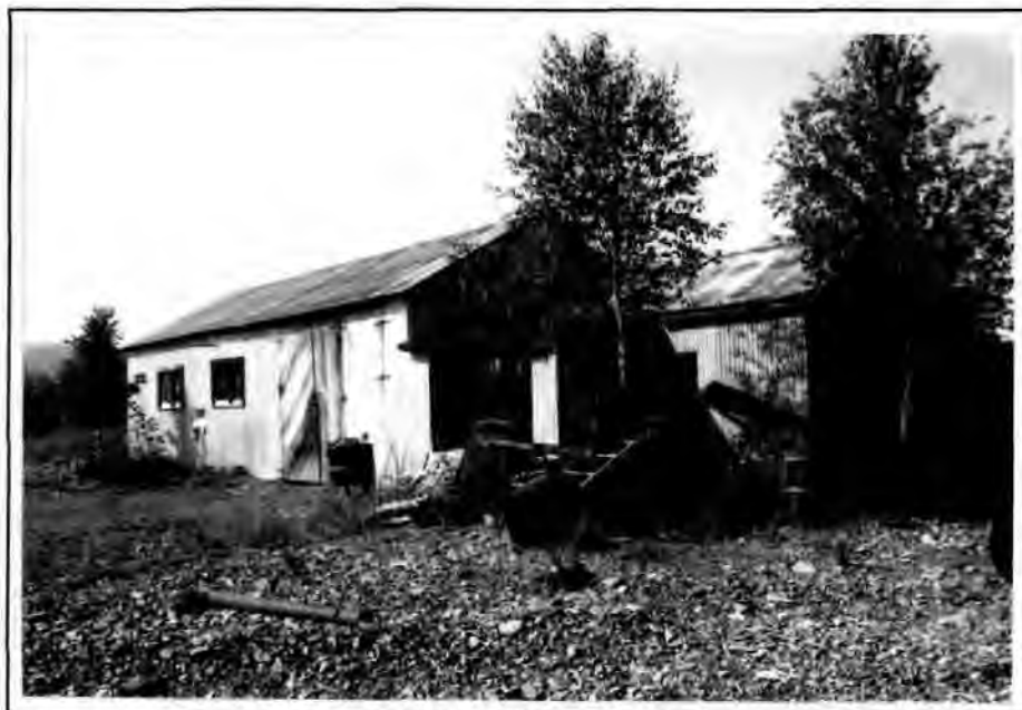
Figure 61. The NADC Machine Shop, 1993. The view is looking northwest.
